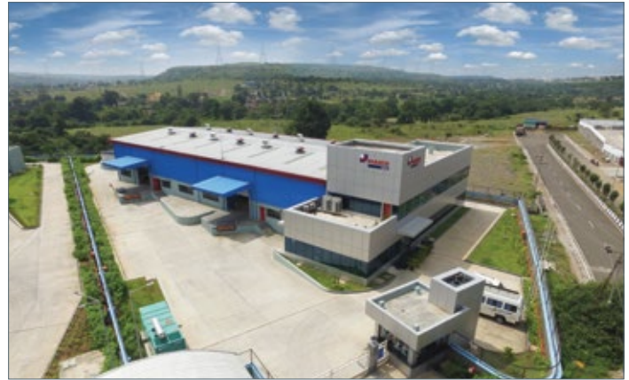
Maico Ventilation Pvt. Ltd is ISO 9001: 2015 company certified.
